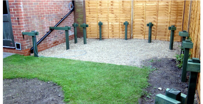
Cross pieces on posts, provide support for longitudinal timbers.
