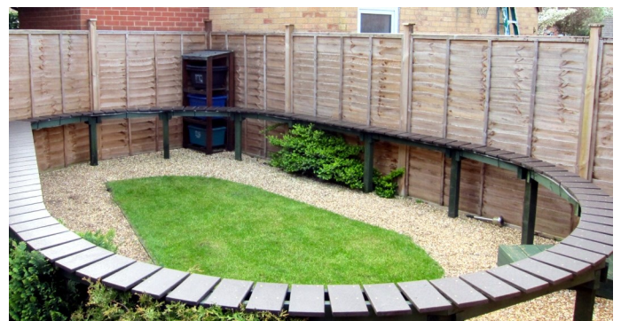
Basic framing and running surface complete.
