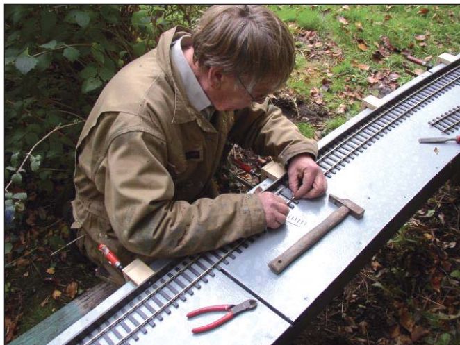
Aksel busy constructing the track.
